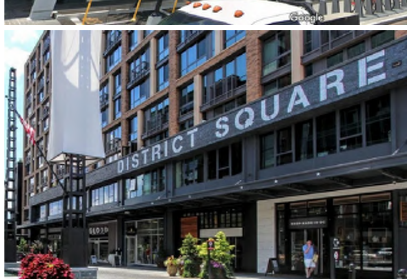
DISTRICT SQUARE, SW
